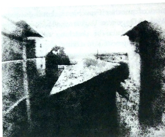
Joseph Nicéphore Niépce. View from His Window at Gras, c. 1826. Heliograph. Niépce produced the world's first photographic image—a view of the courtyard buildings on his estate in about 1826. It was made on a sheet of pewter covered with bitumen of Judea, a kind of asphalt that hardened when exposed to light. The unexposed, still-soft bitumen was then dissolved, leaving a permanent image. The exposure time was so long (eight hours) that the sun moved across the sky and illuminated both sides of the courtyard.
